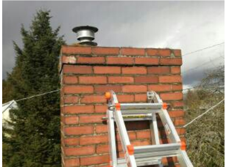
recommend adding chimney cap
